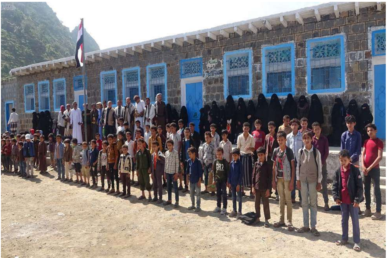
Al-Fawz School in Bani Saeed, Al-Ja'fariya, with four newly built classrooms made of sustainable stone, along with restrooms, improving the school facilities. Photo: AGF
